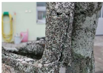
**Crack above corroding reinforcement**
