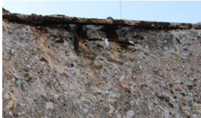
**Massive loss of mass under reinforcement level**
