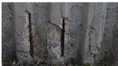
**Massive loss of mass above reinforcement level**
